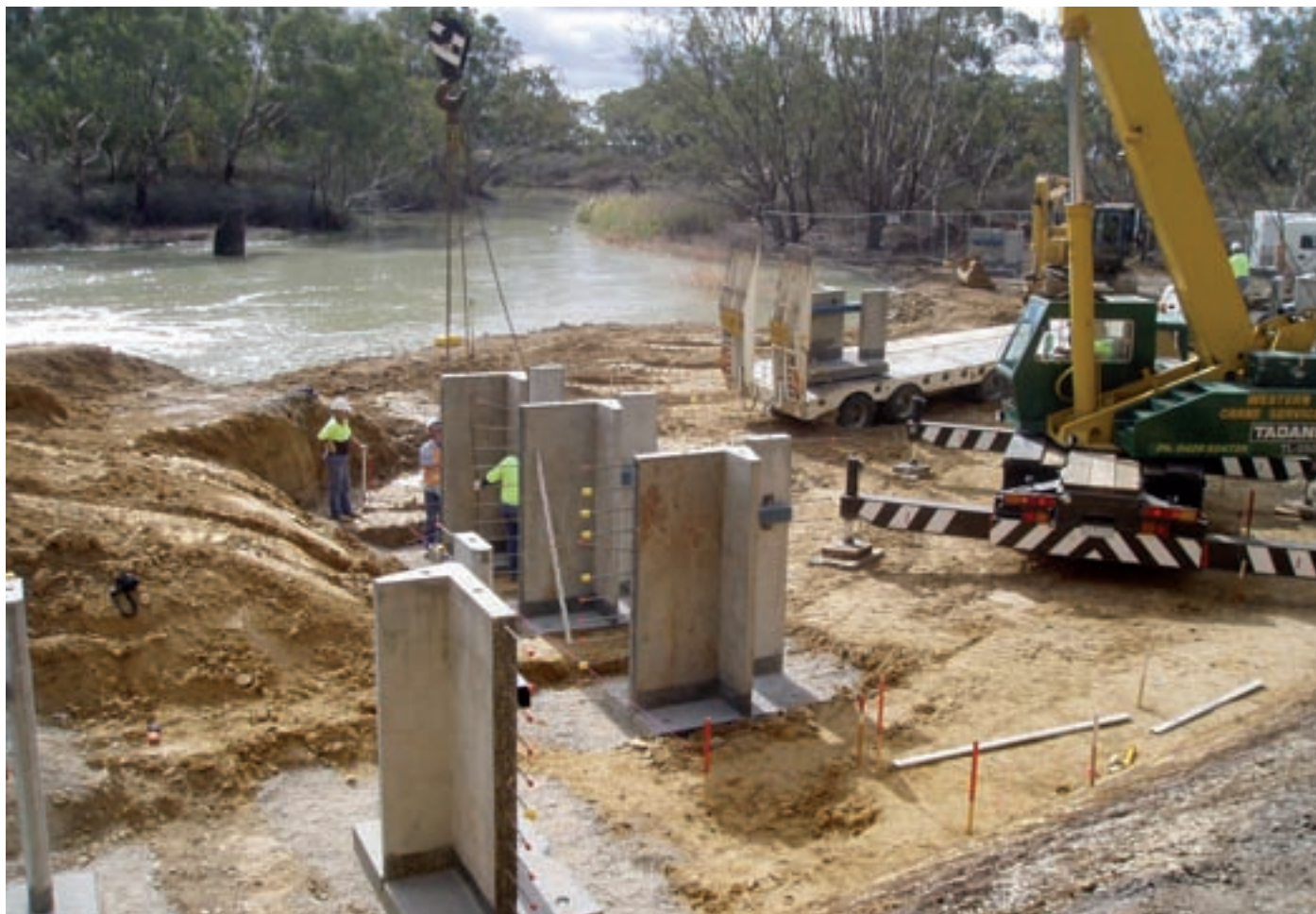
Construction of Kerang Weir Fishway funded by North Central CMA, alongside the Kerang Weir on the Loddon River. The project was completed in 2008/09.
