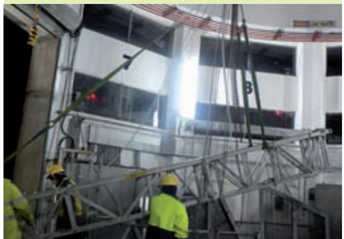
Eildon outlet works
