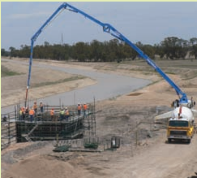
Mokoan Diverters Pump Station concrete pour.
