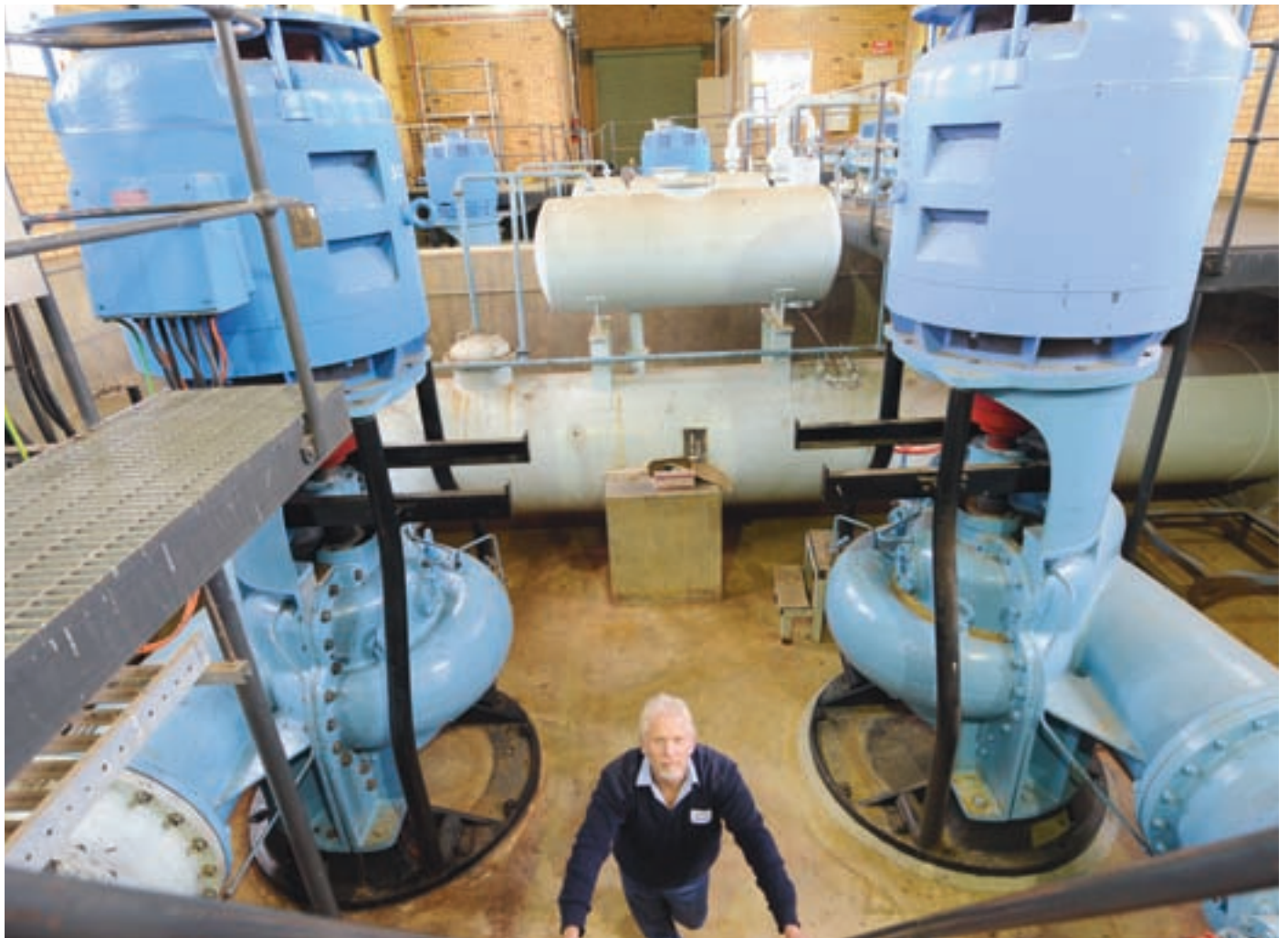
G-MW's Steven Wickham inside the Greens Lake Pump Station in the Rochester-Campaspe Area.
