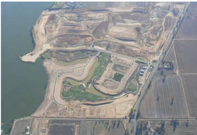
Earthworks for residential development at Silverwoods Estate, Yarrawonga.
