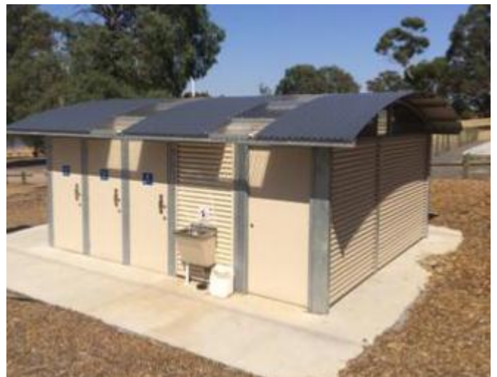
Upgraded toilet facilities at Cairn Curran Reservoir.
