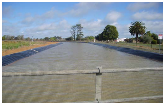
Plastic lined channel at Tongala
